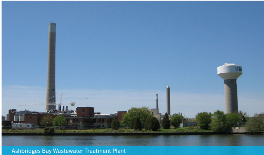
Ashbridges Bay Wastewater Treatment Plant
